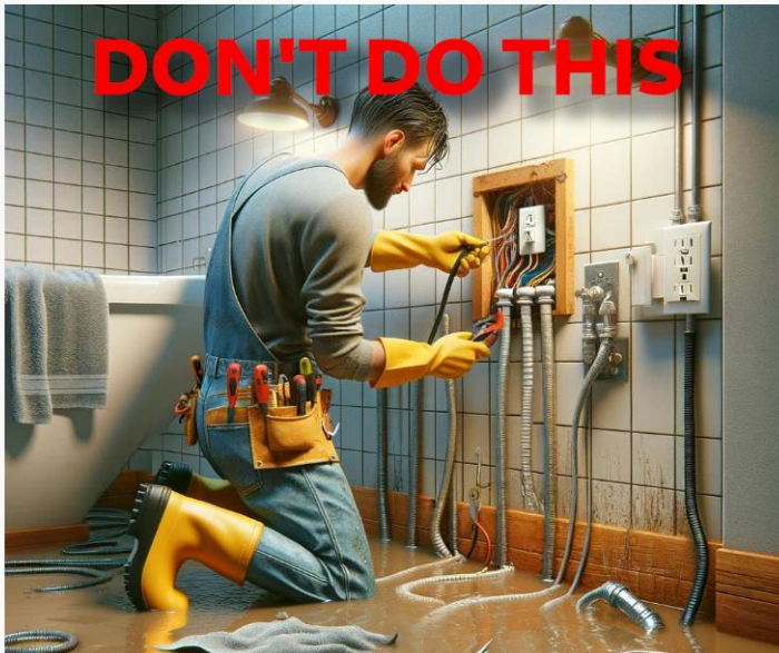
Figure 2 – Never work in wet/moisture rooms
